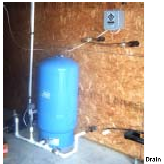
Fig. 1: Free Space to allow for proper backwashing; Anchor 1/2" drain hose from water valve to drain. Water must backwash at 10 gpm. Backpressure from undersized drains must be avoided (well pump to bladder tank shown above, pre-install).
