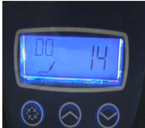
Fig 4 If 2000 gallon backwash isn't reached in certain amount of time, the system will backwash after set amount of days (14 days in Fig 4) regardless of remaining water.
