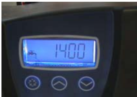
Fig 5 Remaining gallons to backwash. Ecosmarte® Control Valve is displaying the remaining gallons to backwash, as indicated by the red LED display.
